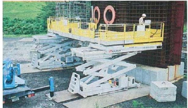
An Automatic Scaffold And Horizontal Rebar Feeding Machine At Kashiwazaki Kariwa-6 In Japan:
