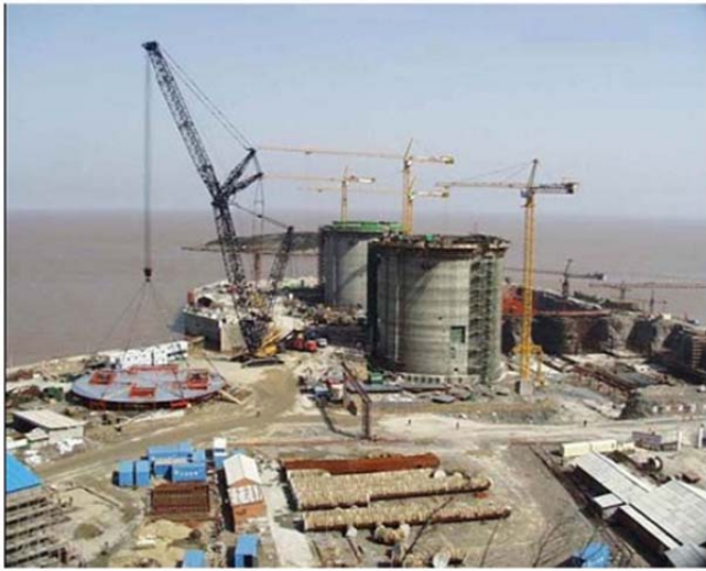
Very Heavy Lift Crane At Qinshan, China:
