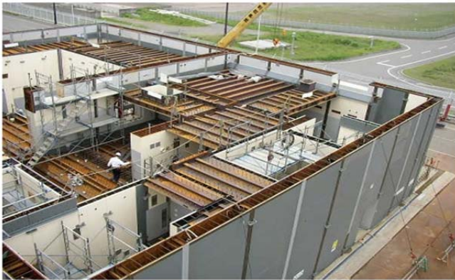
Steel Plate Reinforced Concrete:
